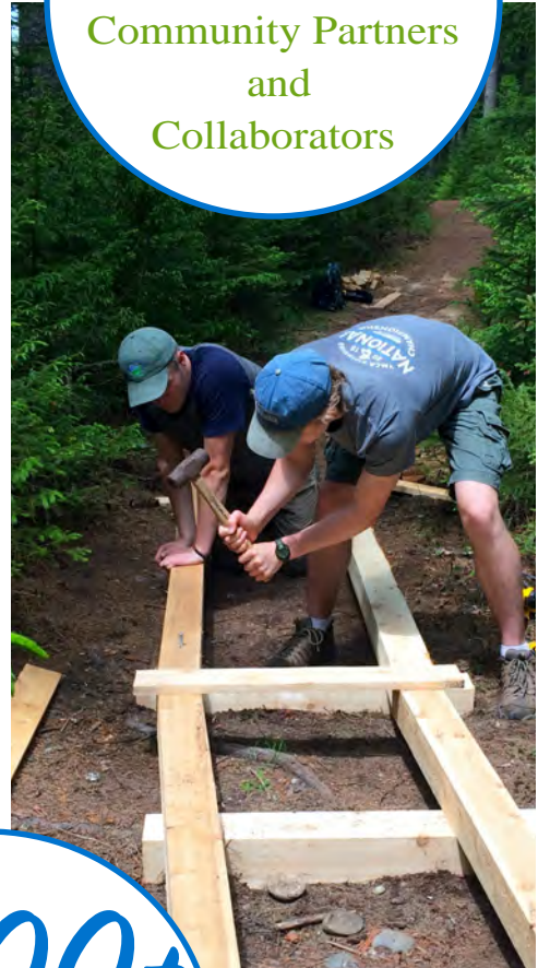
Building new bog bridging at Green Point Preserve in West Bath
